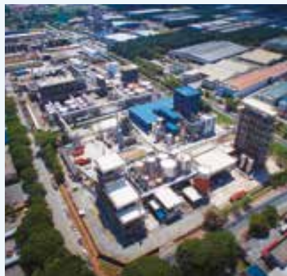
Manufacturing complex, aerial view
