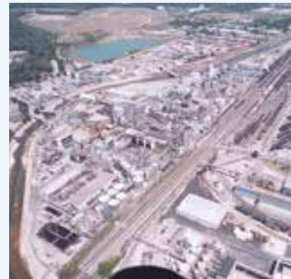
Manufacturing complex, aerial view
