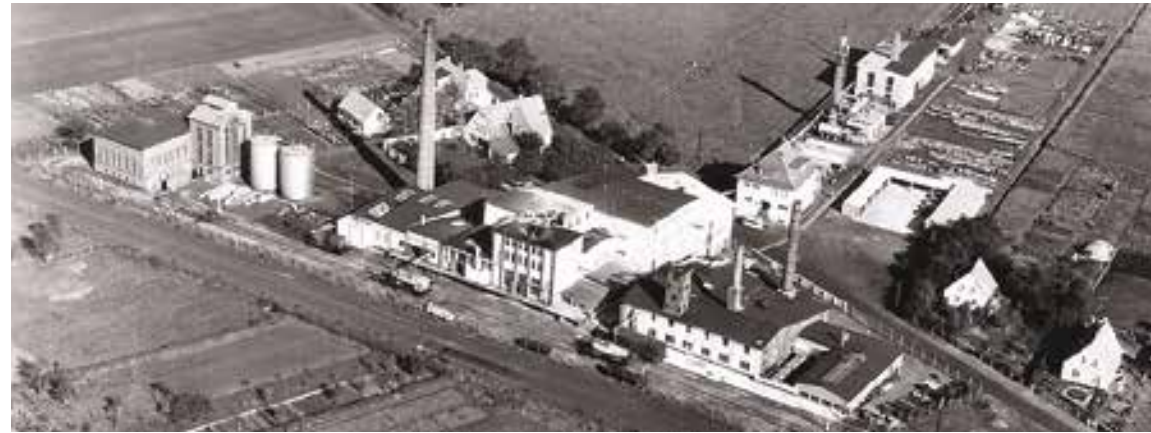
Neynaber Chemie GmbH production site in Loxstedt, Germany
