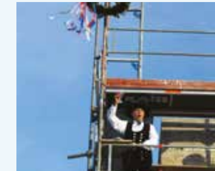
Traditional Roofing-In ceremony of the TDC (2012)
