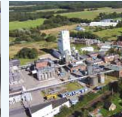
Manufacturing complex, aerial view
